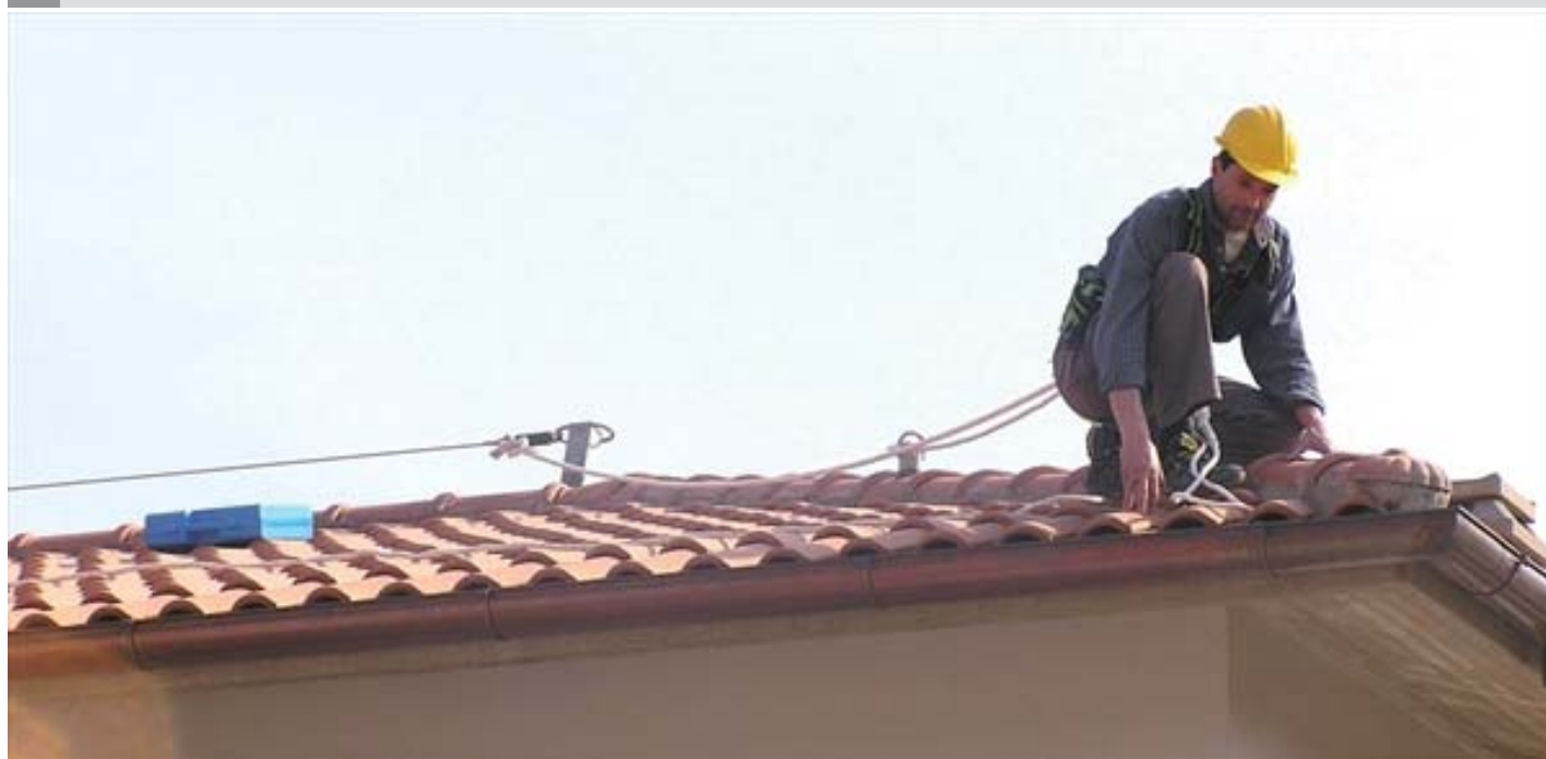
Fig. 2b Safety rope system, gable roof
