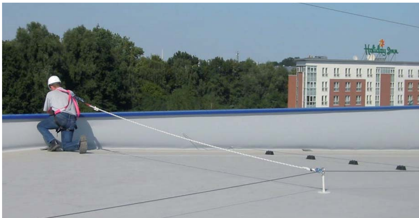
Fig. 2a Safety rope system, flat roof
